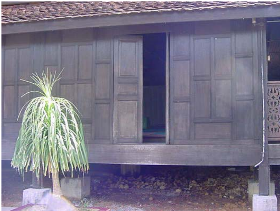
Figure 4: Modular wall's partition with interlocking style.
